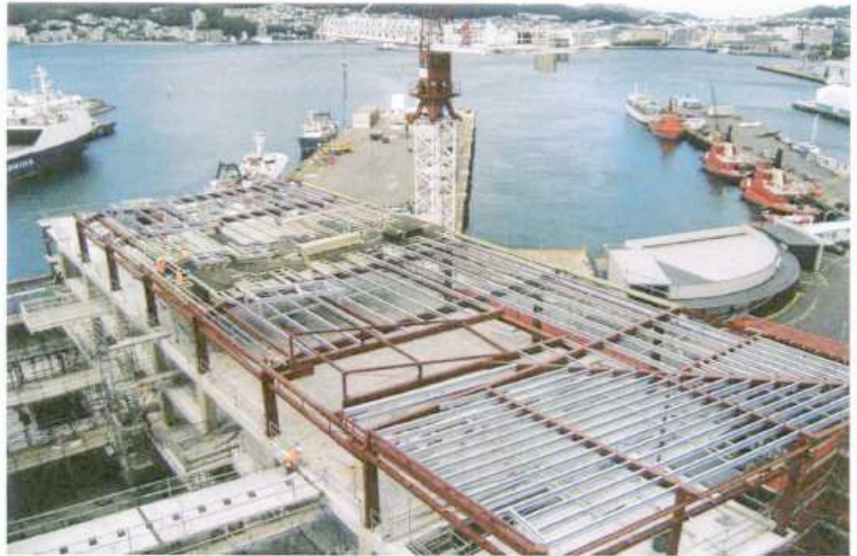
Above: The steelwork for the roofing of one of the piers.
