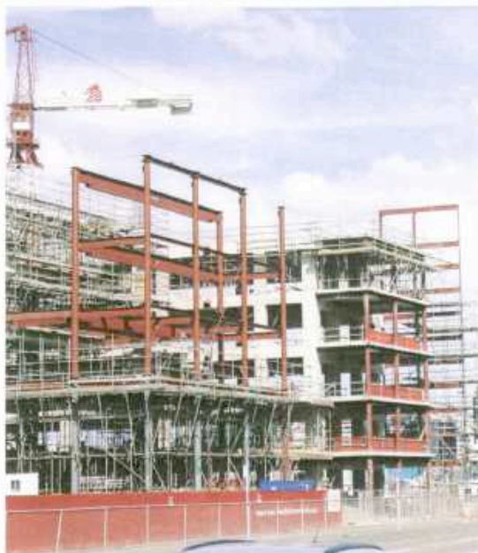
Above: The steel-framed bridges that connect the concrete piers.
