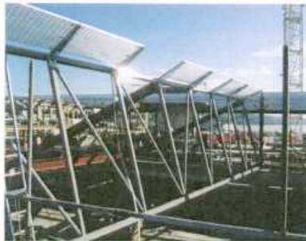
Above: The steelwork for the roofing of one of the piers.
