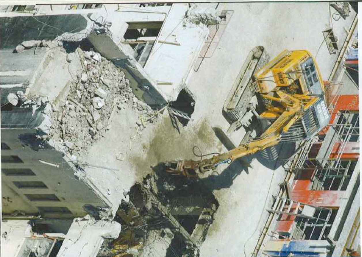
THIS PAGE The demolition process involved craning machinery onto the top of building site; it then works its way down to the ground.
